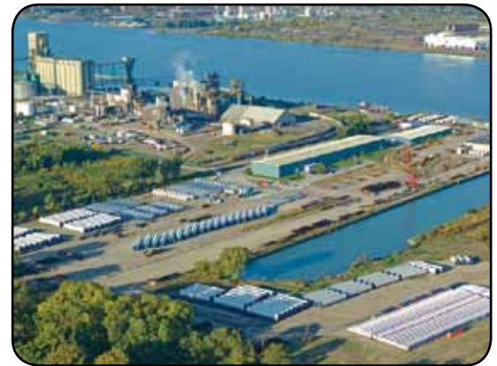
Aerial view of the staging area at Port of Windsor. Photo © Morterm Limited.
